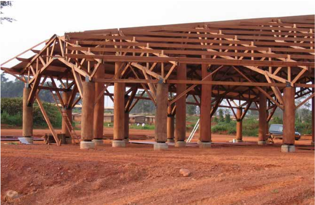
Triangulated structure made of Kosipo with posts made of Tali Built by J.-Y. Riaux (Mindourou, Cameroon) © Jean-Yves Riaux (photo from the Atlas of Tropical Timbers, 2016)
