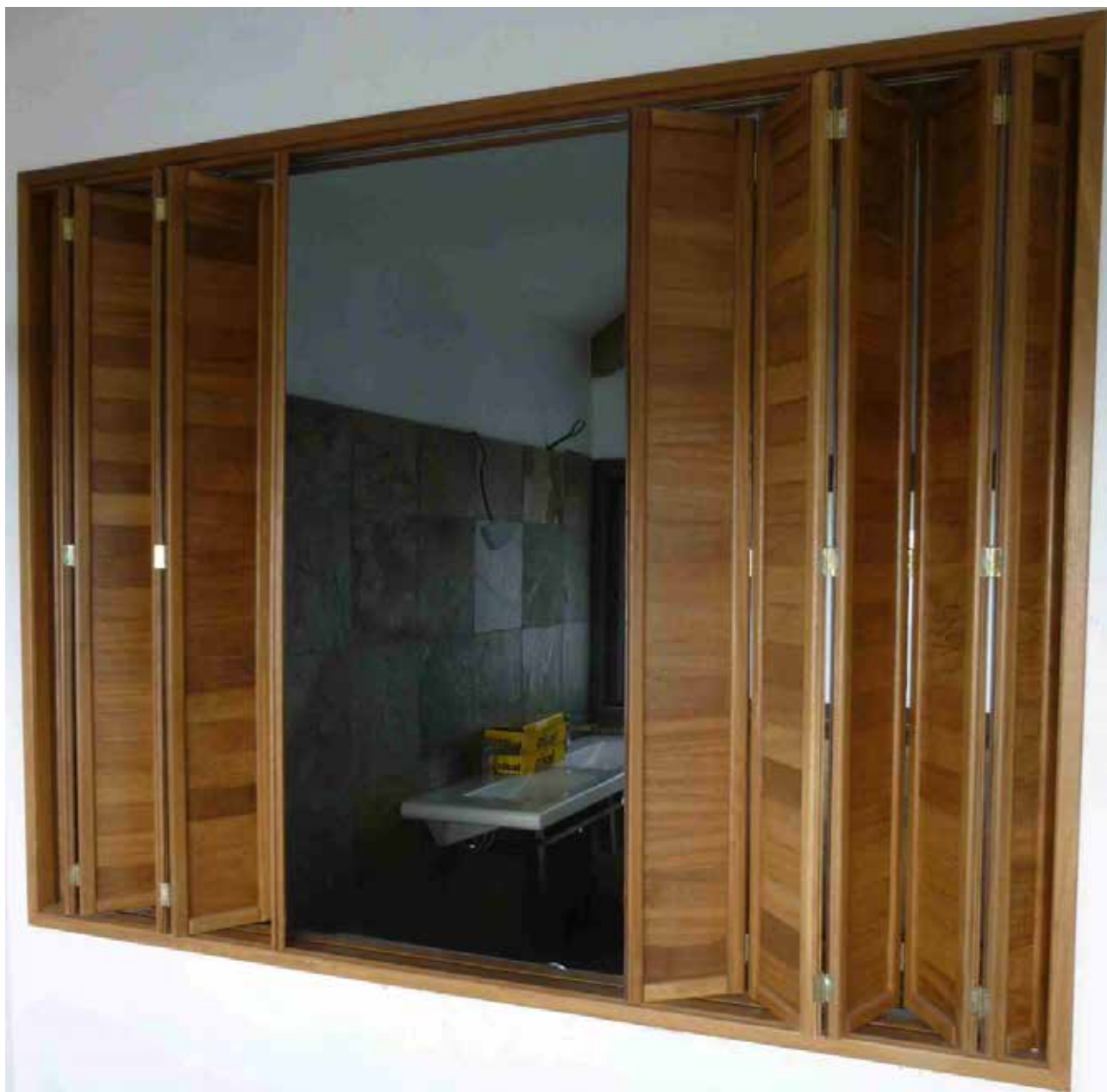
Folding shutter made using Movingui Fibres Industries Bois , La Réunion
