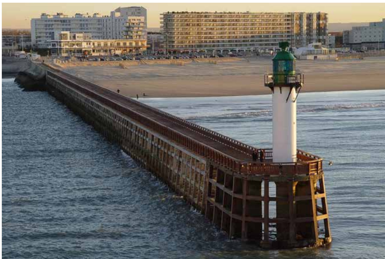
Decking of the Calais jetty in Azobé – Completed by Bois et Loisirs, France © Denis Delequeuche, Bois et Loisirs (photo from the Tropical Timber Atlas 2016 )
