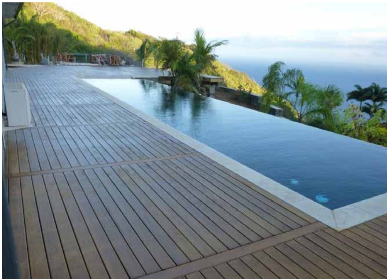
Osanga decking bordering an infinity pool – Supplies by Fibres Industries Bois , Made by Agencement Tiby , La Réunion (France). © David Bodelu, Fibres Industries Bois (photo extracted from the Atlas of Tropical Timbers 2016 99 ).
