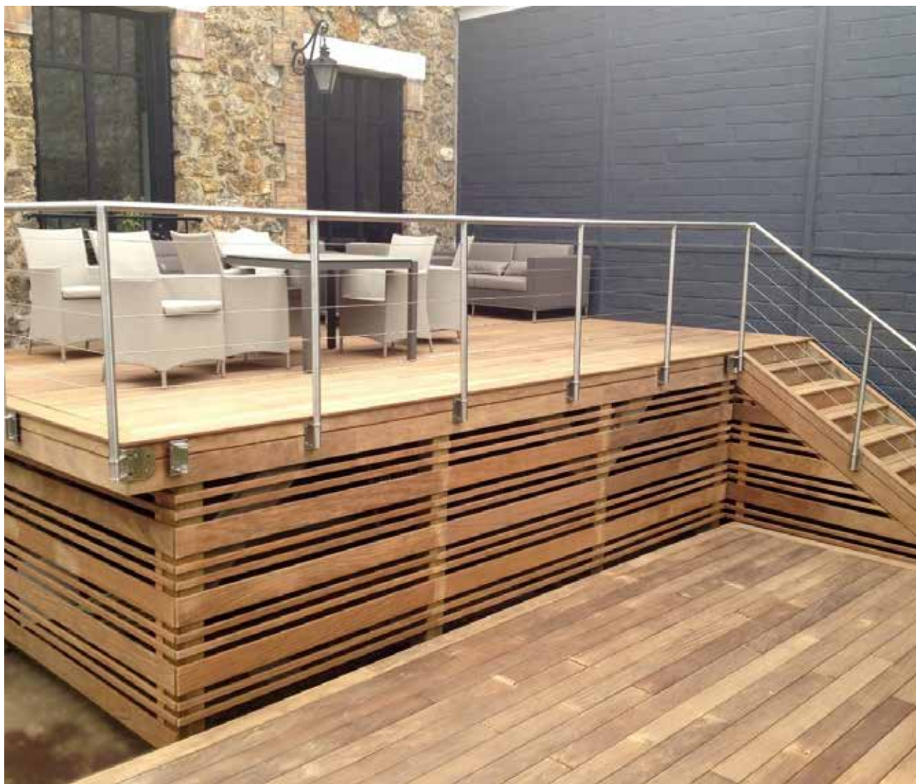
Elevated staircase and decking made of Afrormosia – Created by Terrasse Nature, Antony (France). © Terrasse Nature (photo from the Tropical Timber Atlas 2016 ).
