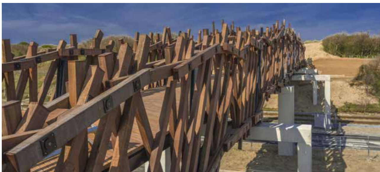
«Het Wrakhout» bridge and its guardrail (Azobé, Okan, and Tali), connected to a bike path and a pedestrian walkway – Welduine, Belgium © van Wijma Kampen
