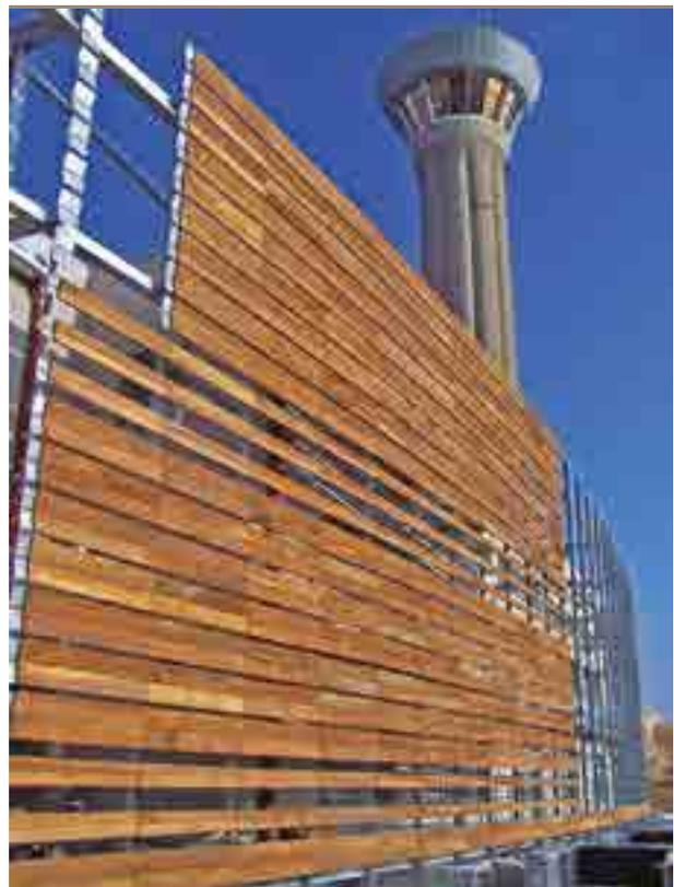
▲ Photo 39: Solar shading façade made with Iroko © M.Vernay
