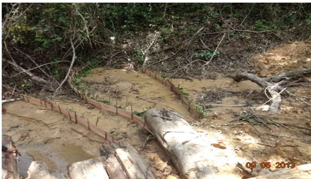
Photo 2 – Riverbank and watercourse stabilisation strips
