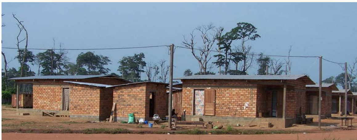
Cabins built at the Ngombé living camp © Antoine COUTURIER
