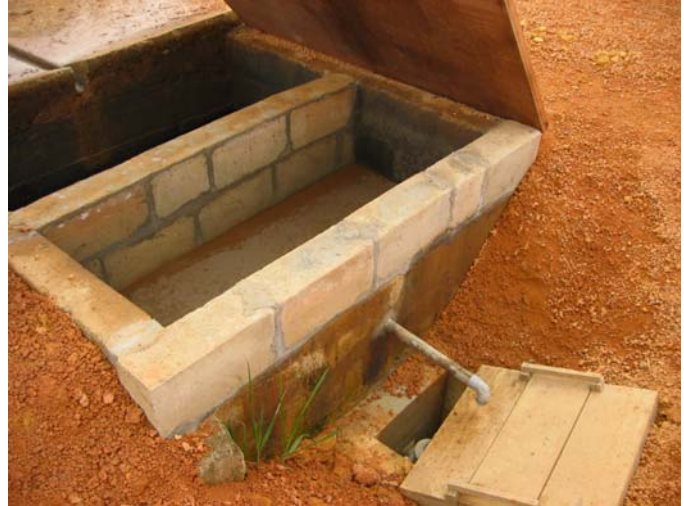
De-silting and hydrocarbon separation tank © Bernard CASSAGNE
