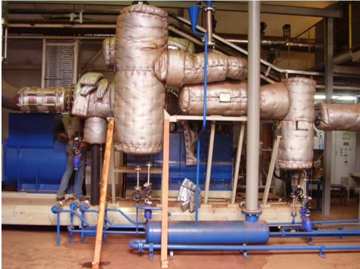
Steam engine installed to generate electricity © IFO
